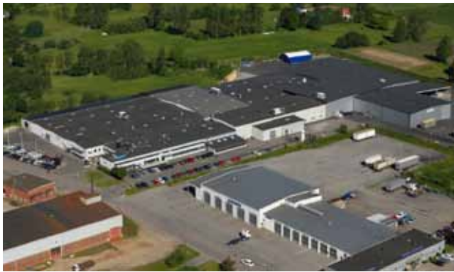
Swegon Tomelilla, Sweden, air diffusers and flow control.
