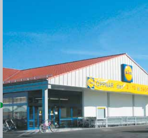
▶ Lidl, Sweden, Norway, Finland, Denmark Air handling units, Air distribution products
