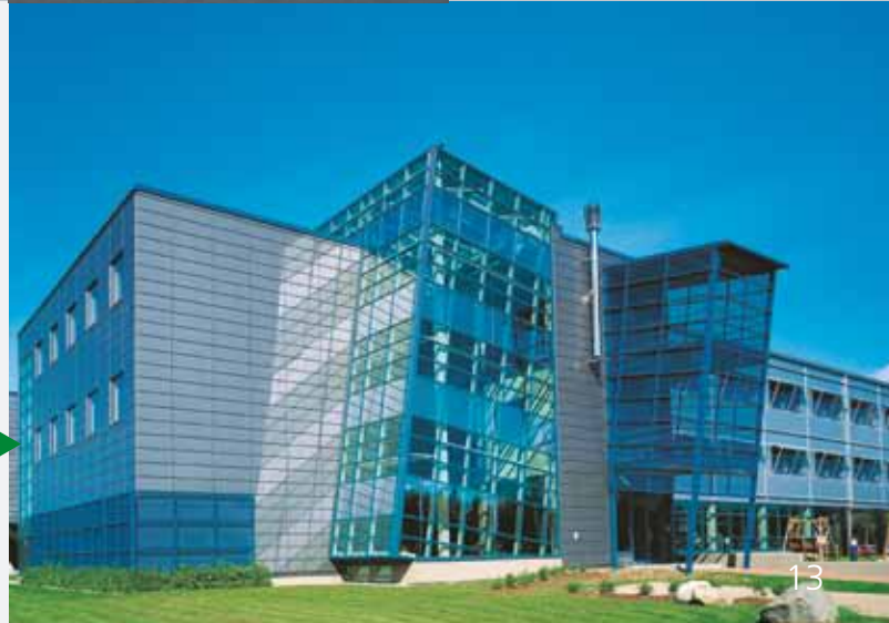
Nokia, Oulu, Finland Air handling units
