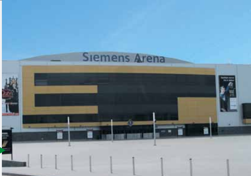
Siemens Arena, Vilnius, Lithuania ▶ Air handling units
